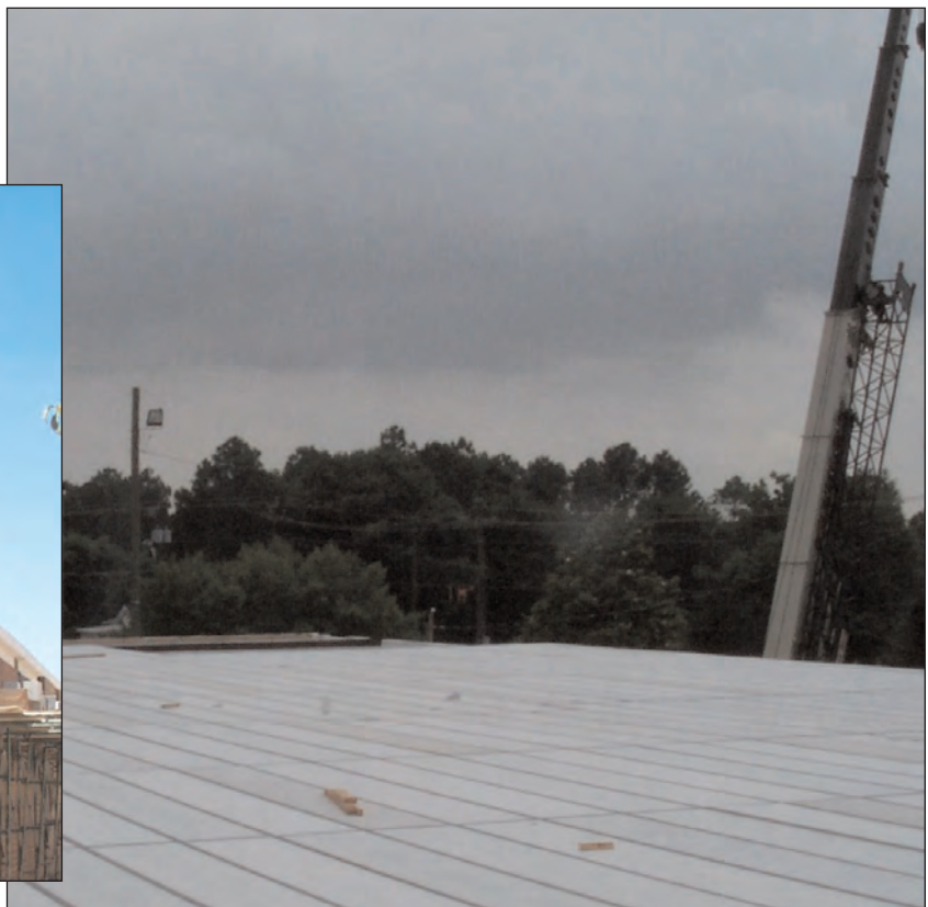
Horizontal (flat) roof panel installation.
