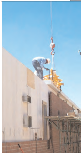
Horizontal (flat) roof panel installation.
