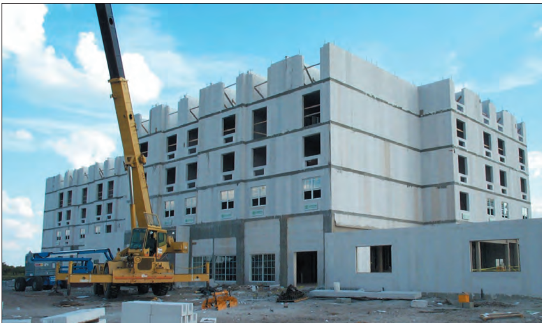
Hotel being constructed of AERCON load bearing vertical wall panels.
