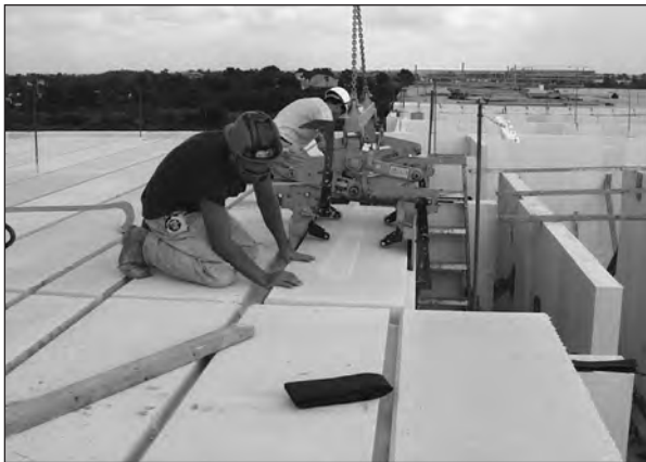
AERCON Floor/Roof Panel Installation
