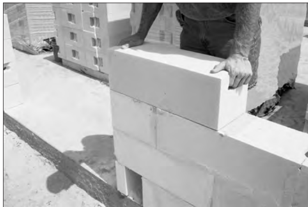
AERCON Block Installation
