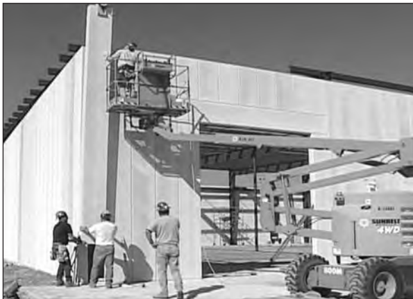
AERCON Non-load Bearing Vertical Wall Panel Installation
