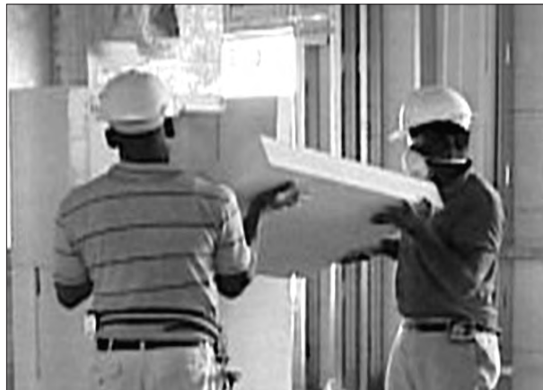
AERCON ValuBlock Installation
