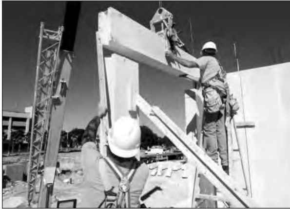
AERCON Lintel and Load Bearing Wall Panel Installation
