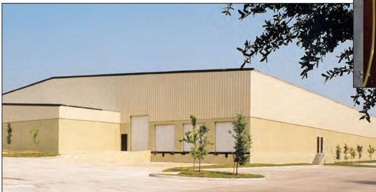
AERCON panels are perfect for this non-load bearing cladding application where the panels are attached to a steel structure.
