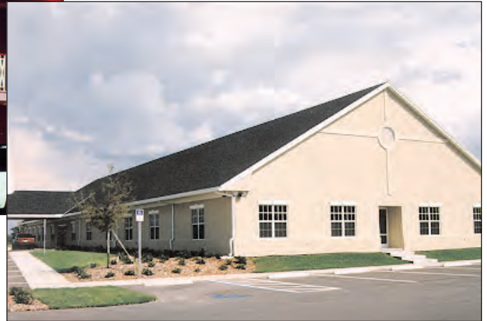
Load bearing vertical wall panels were chosen for this beautiful Central Florida Church.
