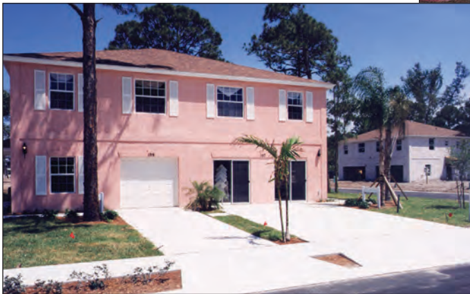
The sound absorption qualities of AERCON allows the two-family occupants of this townhouse maximum privacy in a small space.
