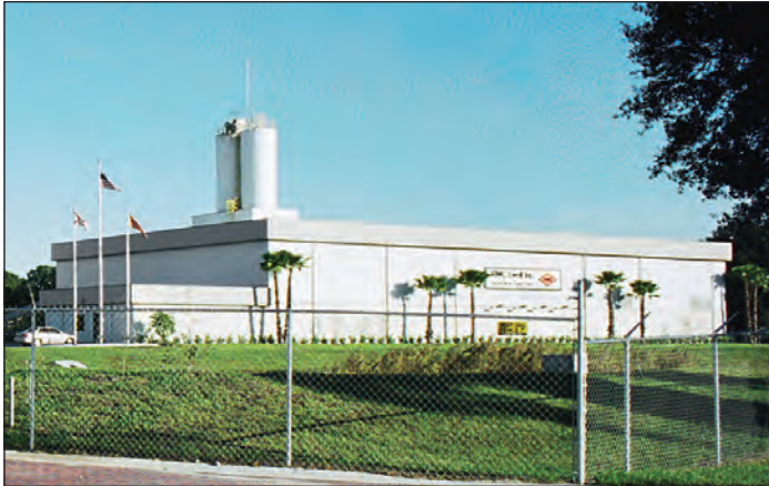
AERCON block was used to build this ultra-modern concrete paver plant facility.
