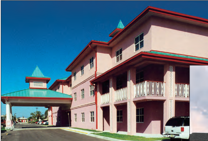
AERCON wall and floor panels were used in the construction of this $4 million, 84-suite hotel expansion.
