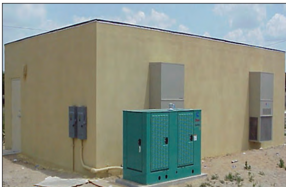
A telecommunications company chose AERCON's energy efficient wall panels for several Communication Equipment Buildings in order to lower their operating costs.
