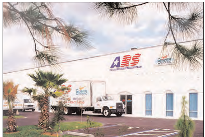
Needing climate-controlled space for sensitive electrical equipment storage, this warehouse owner chose AERCON for its superior thermal insulation.
