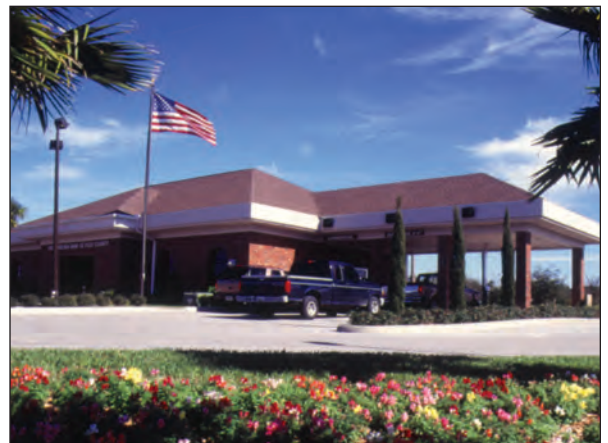
10" AERCON block was used to build this bank building.
