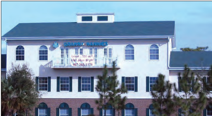
This office building used AERCON load bearing wall panels and floor panels in conjunction with structural steel framing.
