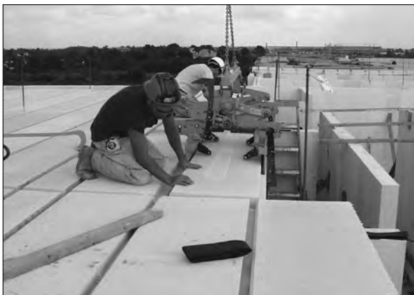
AERCON Floor/Roof Panel Installation
