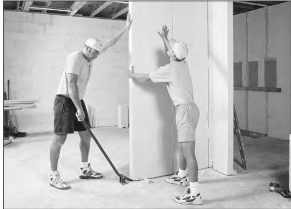
AERCON Interior Wall Partition Installation
