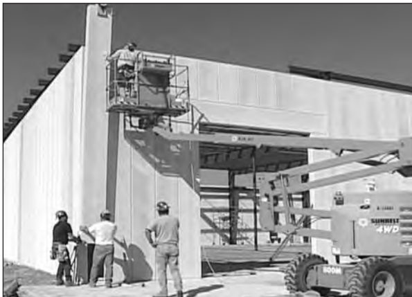
AERCON Non-load Bearing Vertical Wall Panel Installation
